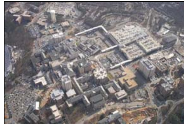
Aerial Photo showing recent construction on UNC Campus
