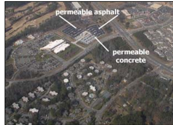
Aerial of Sample Campus Parking Lot
