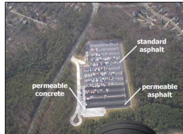
Aerial of Sample Campus Parking Lot
