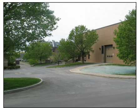
Figure 20. The current service entry to the Food Sciences Complex off of Judd Falls Road
