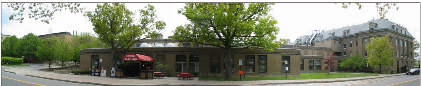
Figure 6. Composite photo of north facade of the Food Science Lab, Stocking Runway, and Stocking Tower along Tower Road
